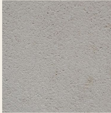
BALD. PROM. MC-411 SANDBLASTING
