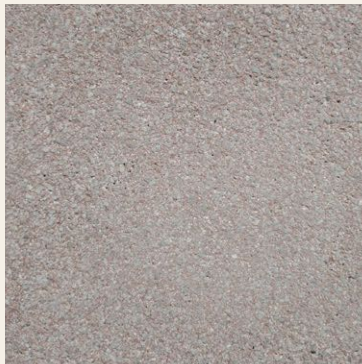
BALD. PROM. N-11 SANDBLASTING
